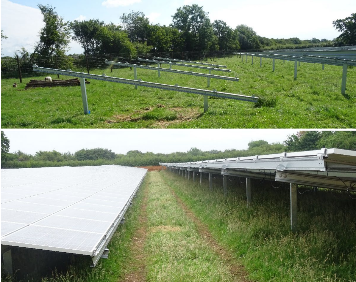
Photos 18 and 19: Panels Under Construction
